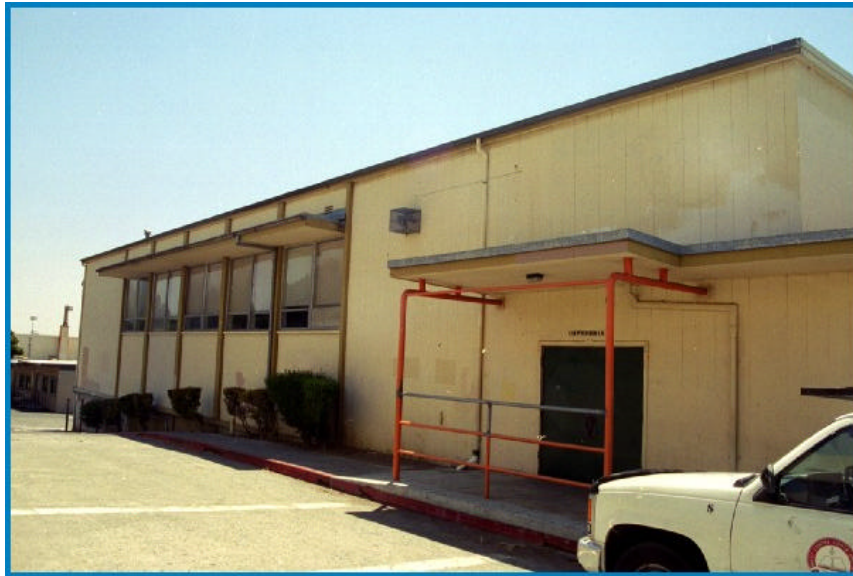
Figure 12: Unit D, Cafeteria, North Elevation
