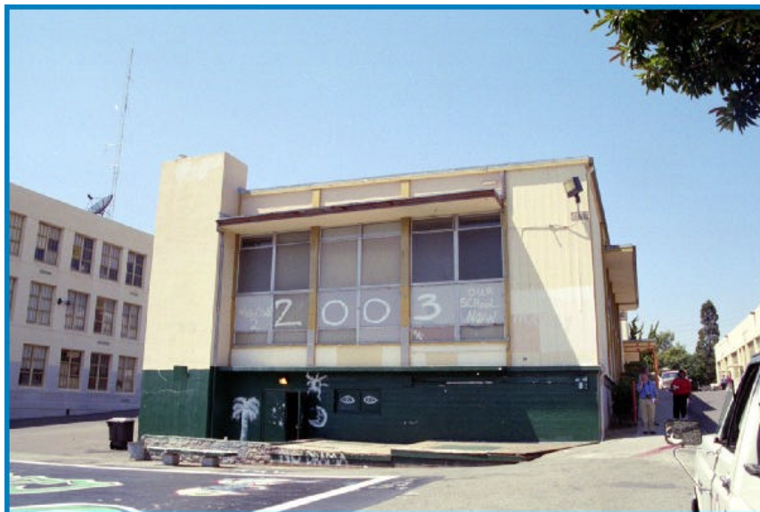
Figure 11: Unit D, Cafeteria, South Elevation
