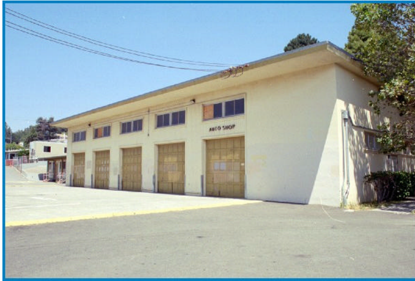
Figure 20: Unit H, Automobile Shop Building, West Elevation
