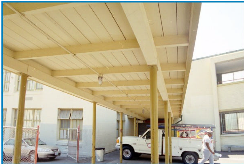
Figure 13: Covered Walkway from Unit D to Unit A
