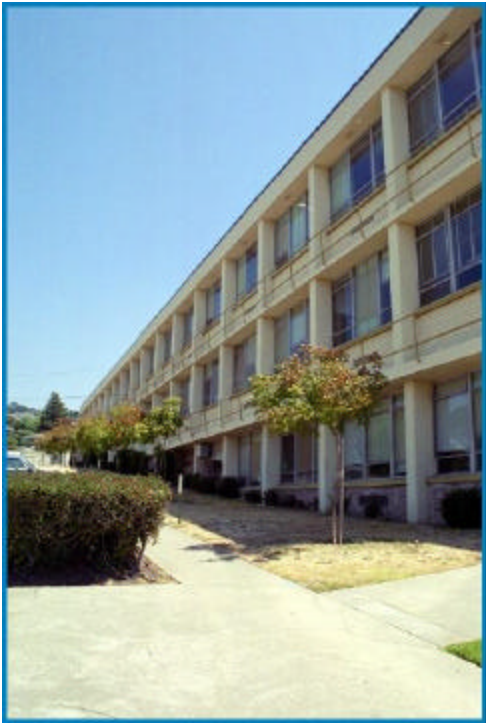
Figure 7: Unit C, Classroom Building, North Elevation
