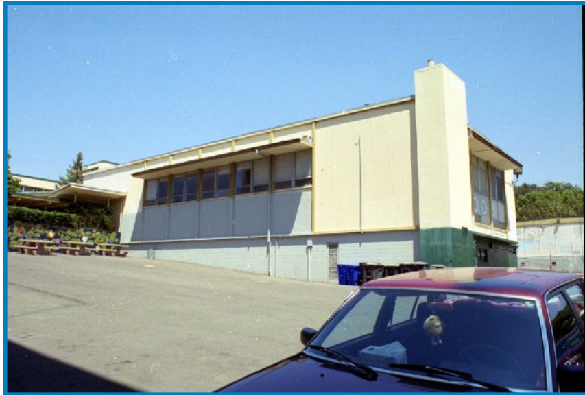
Figure 10: Unit D, Cafeteria, West Elevation
