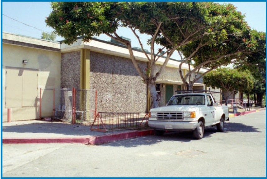
Figure 18: Unit F, Drama and Music Building, West Elevation
