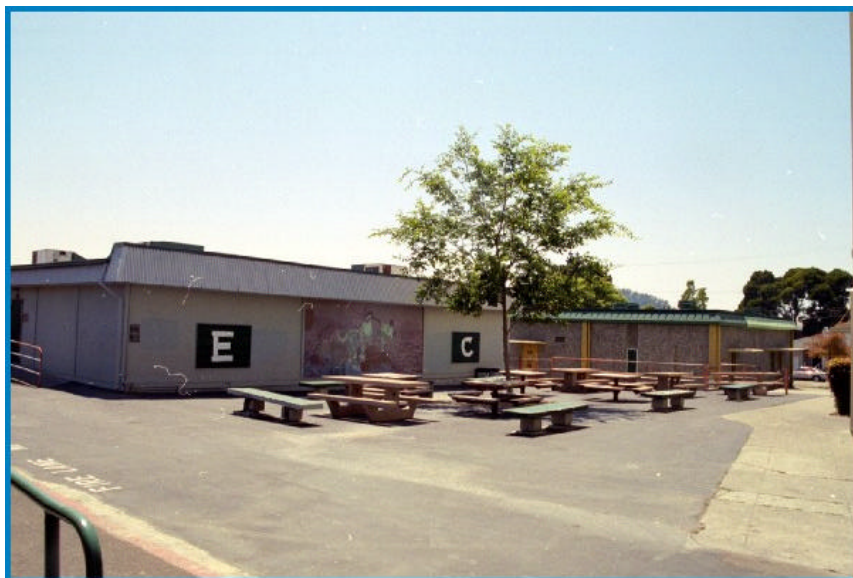
Figure 17: Unit E, Gymnasium Locker Addition, North Elevation, Unit B, Science Building beyond
