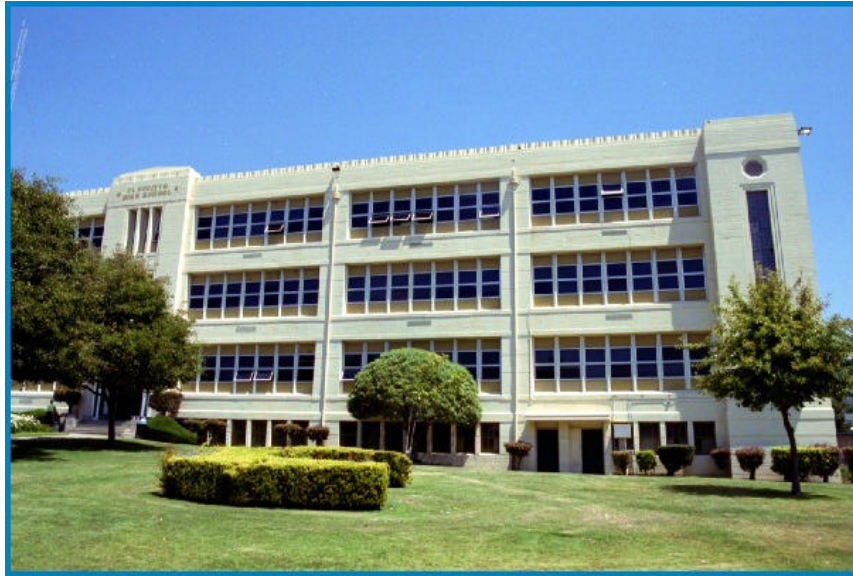
Figure 2: Unit A, Main Classroom Building
